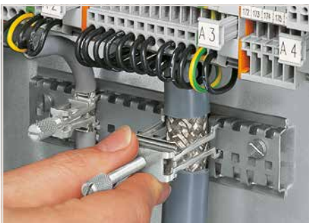
Securing an additional shield clamping saddle.
