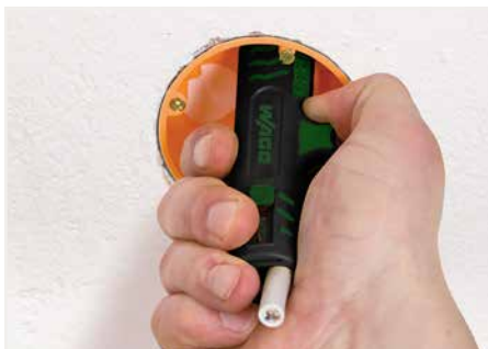
Stripping a cable sheath.
