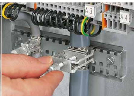
Tightening/removing a shield clamping saddle.
