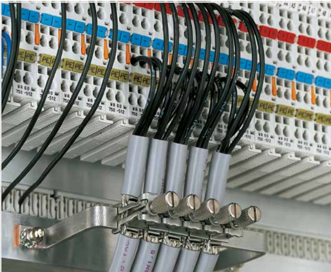
U-shaped (10 x 3) mm copper busbar
