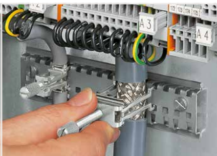
Securing an additional shield clamping saddle.
