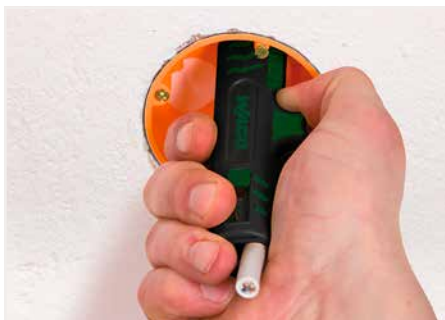
Stripping a cable sheath.
