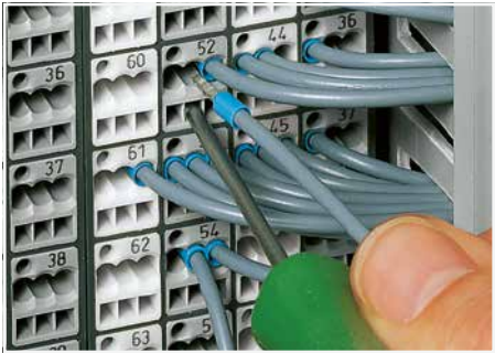
Terminating ferruled conductors via operating tool.
