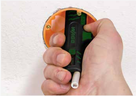
Stripping a cable sheath.
