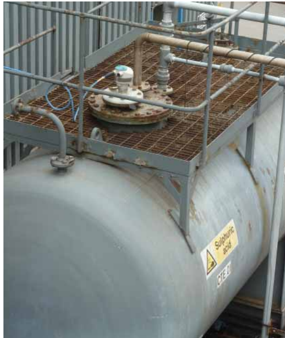
Installation of the SITRANS LR250 Threaded PVDF Antenna.
